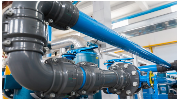
Elbows, Connectors, Butterfly Valves, and Aluminum Piping
